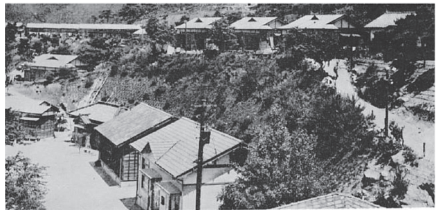
十坪患者住宅(千代田寮附近) 10 tsubo Cottages of couples (360 square feet house).
