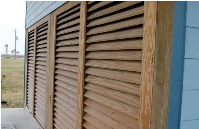
Wood louvers installed beneath an elevated house in a V zone are a good alternative to solid breakaway walls
