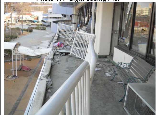
Photo 19: Damage on the second floor deck
