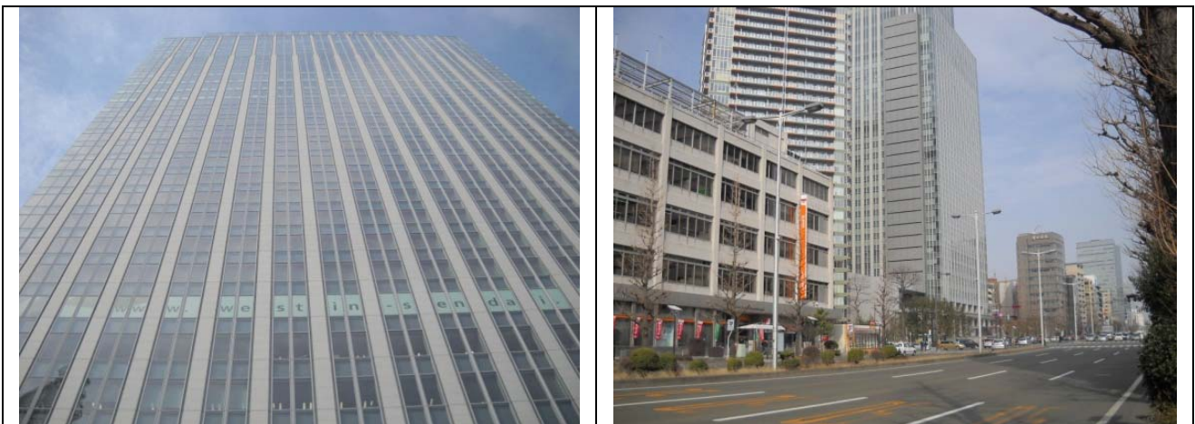
Photo 1: a 37-story and a 29-story office building in Sendai without structural damage
