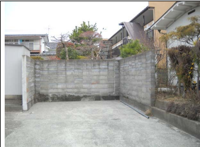
Photo 6: Concrete block walls (Undamaged)
