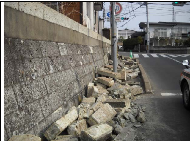
Photo 8: Fall of tuff masonry walls
