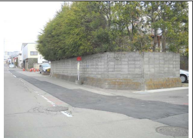
Photo 7: Concrete Block walls (Undamaged)
