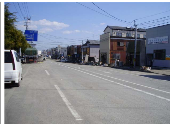
Photo 5: Damaged area of Shiogama City
