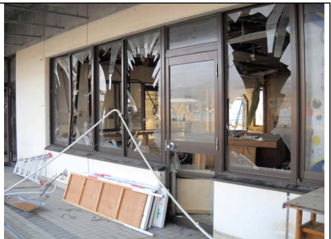
Photo 18: Tsunami Damage in the first Story
