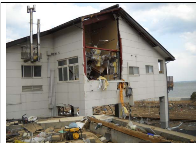
Photo 11: Damage by tsunami wave
