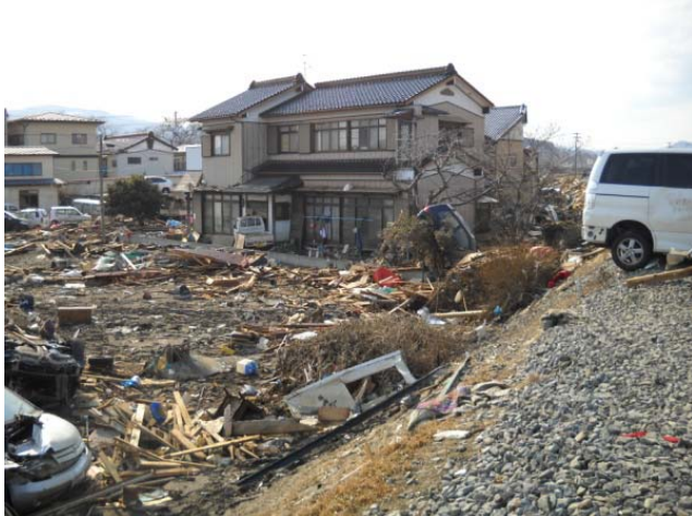
Photo 23: Tsunami wave crossed the railway line
