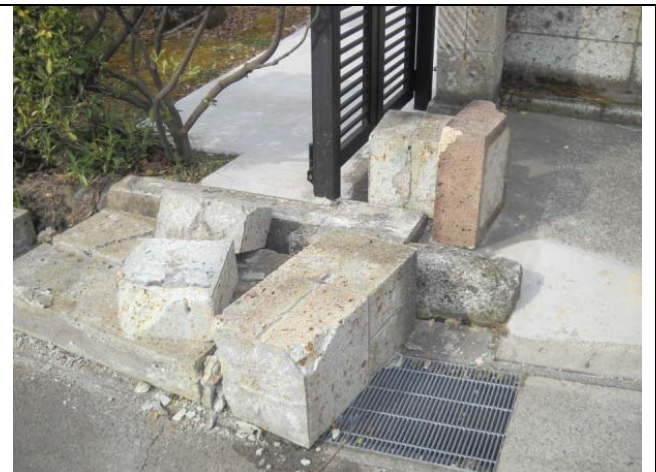
Photo 9: Damage of tuff masonry walls
