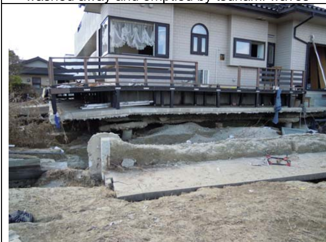
Photo 5: Foundation was exposed by tsunami wave wash
