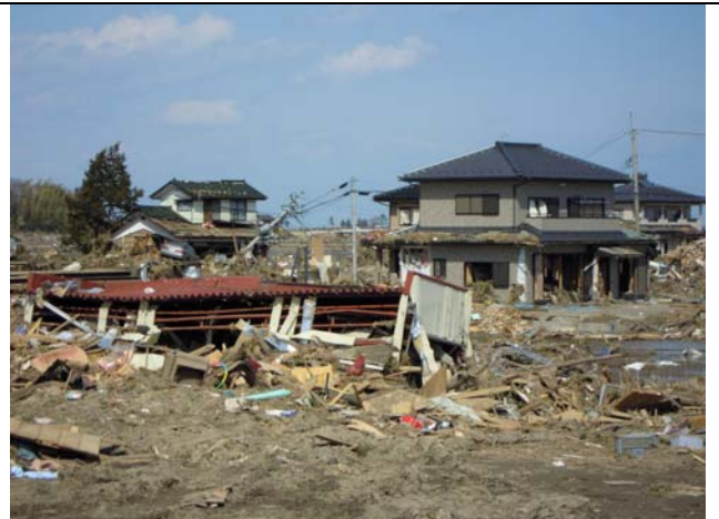
Photo 12: Tsunami water reached the first story roof
