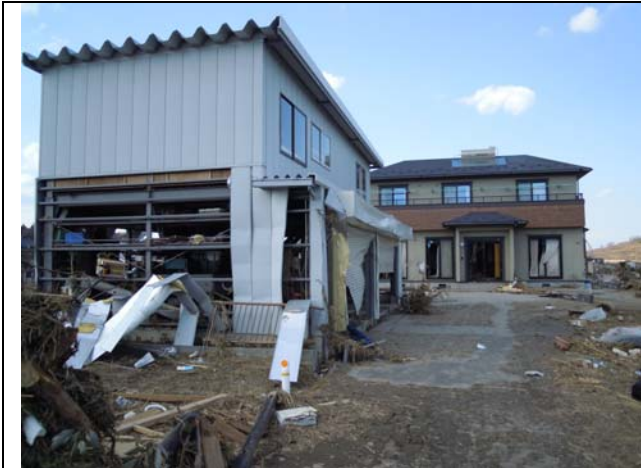
Photo 9: Exterior walls were broken and water got inside by tsunami attacks
