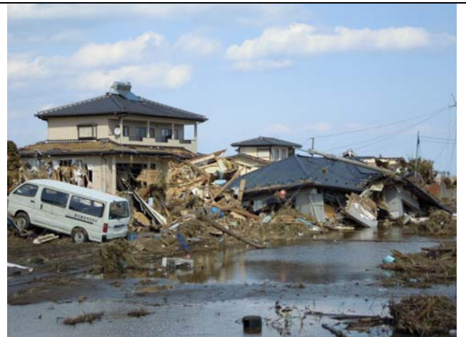
Photo 2: Tsunami wave reached the roof of the first story of this house
