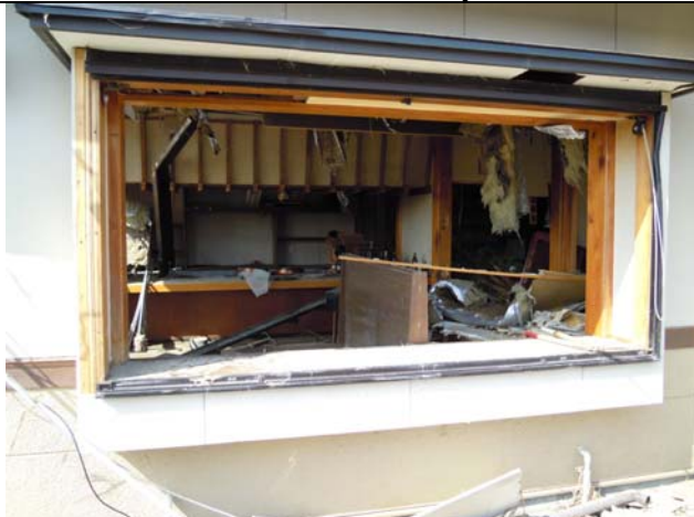
Photo 13: The inside of a house after tsunami attack. No furniture is left in the house.
