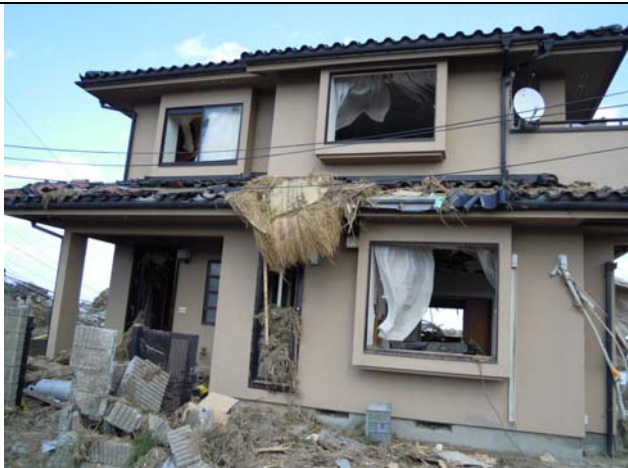
Photo 11: Tsunami water reached the first story roof, and concrete block masonry walls fell down
