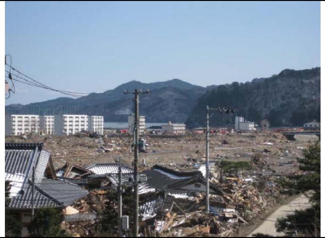
Photo 4: Only RC buildings are standing (previously Housing for Employment Promotion)
