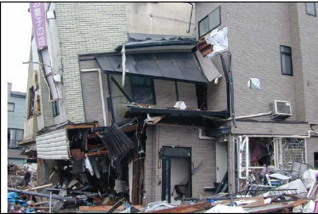
Photo 4: The first story of a timber house was washed away and the second story is about to collapse. The building behind is steel construction
