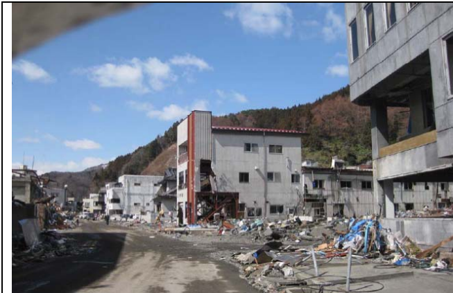
Photo 6: RC and steel buildings, exterior finishing fell from the steel building
