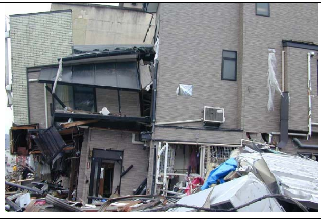
Photo 4: The first story of a timber house was washed away and the second story is about to collapse. The building behind is steel construction
