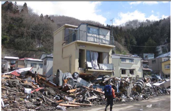
Photo 4: Only RC or concrete block masonry buildings are standing
