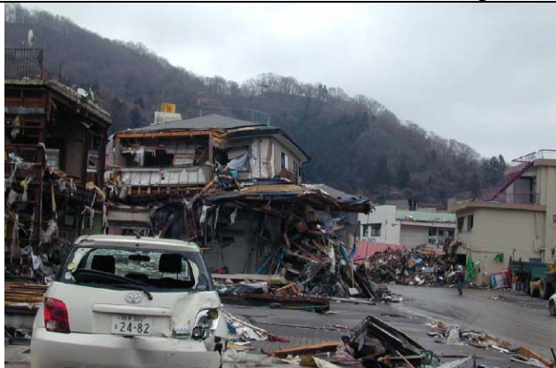
Photo 5: Timber and steel construction suffered more significant damage. RC buildings on the coast side suffered less damage.
