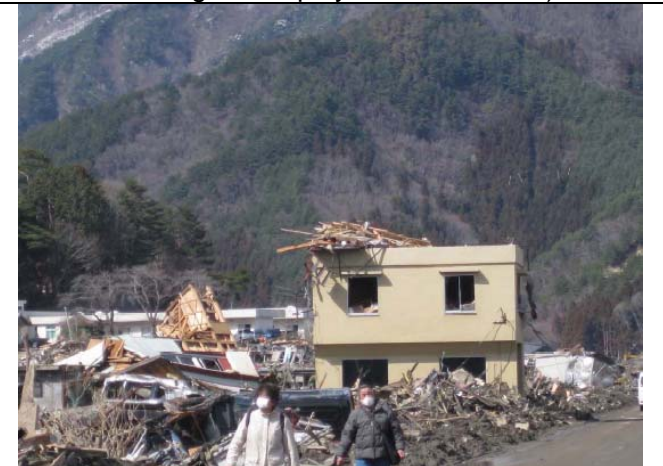
Photo 6: RC or concrete block masonry buildings are left standing
