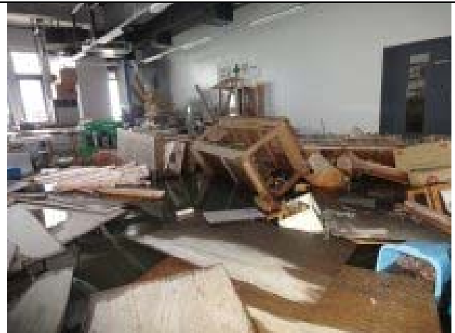
Photo 14: Damage of a technical training building
