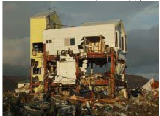
Photo 42: Minami-hama area; a steel construction
