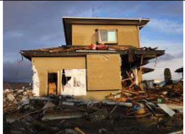
Photo 44: Minami-hama area; a timber house standing (1)
