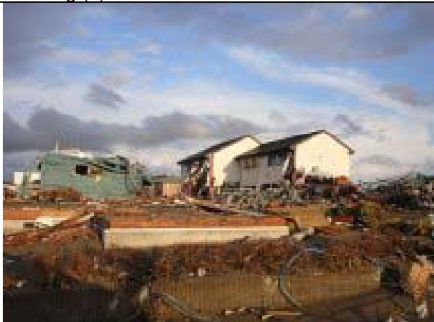
Photo 47: Minami-hama area; steel construction
