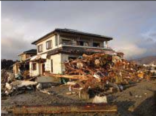
Photo 45: Minami-hama area; a timber house standing (2)
