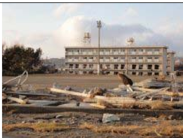
Photo 50: Minami-hama area; Minami-hama apartment building
