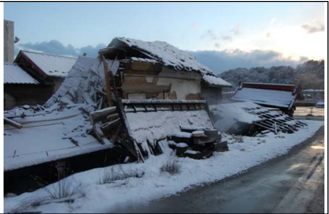
Photo 4: A collapsed house near Myoujin Bridge of the Takagi River
