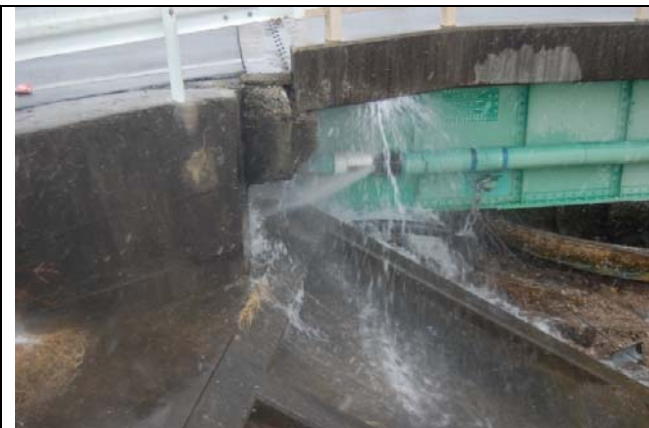
Photo 1: Matshima bridge on the Takagi River. Leakage of city water from water pipes.
