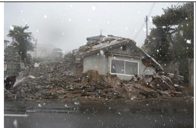
Photo 2: Collapse of a vacant house at Takagi
