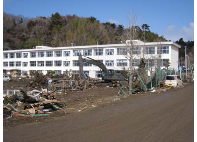
Photo 2: Overall view of Nobiru Elementary School, retrofitted.
