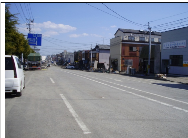
Photo 5: Damaged area of Shiogama City
