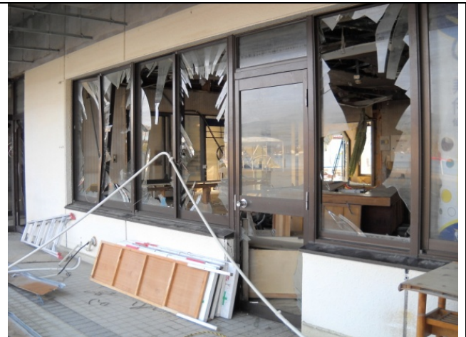
Photo 18: Tsunami Damage in the first Story
