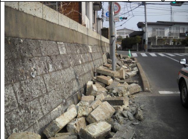
Photo 8: Fall of tuff masonry walls
