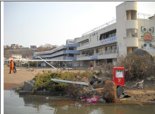
Photo 17: “Sight-seeing Pier (Ocean View Building)”
