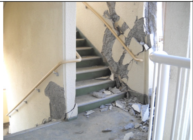
Photo 20: Damage on staircase landing
