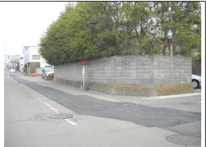
Photo 7: Concrete Block walls (Undamaged)
