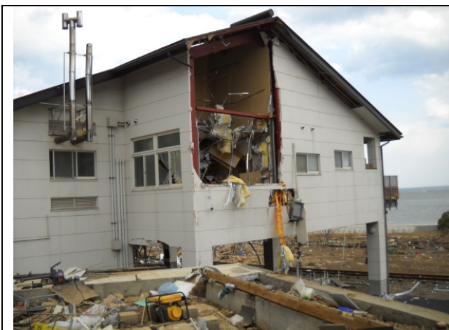
Photo 11: Damage by tsunami wave
