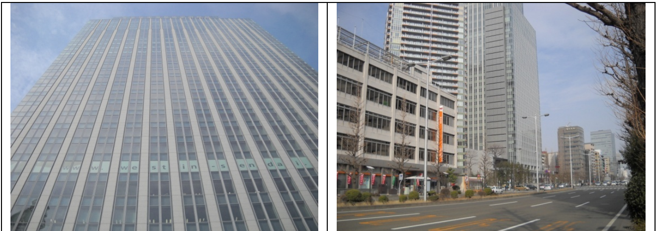
Photo 1: a 37-story office building and a 29-story office building in Sendai without structural damage
