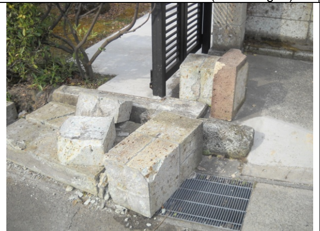
Photo 9: Damage of tuff masonry walls
