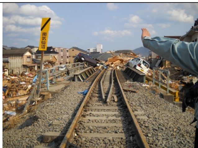
Photo 22: Damage on railway of the Kesenuma Line
