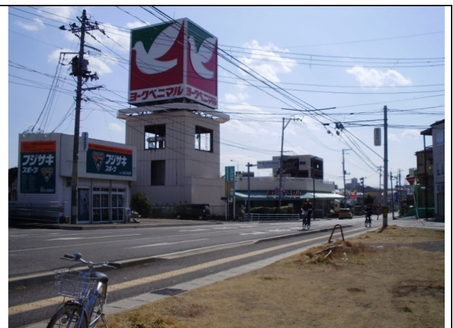
Photo 6: Undamaged area of Shiogama City
