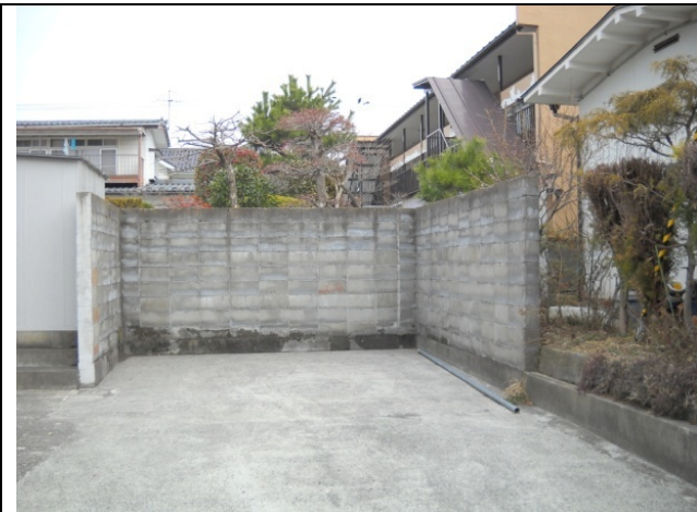
Photo 6: Concrete block walls (Undamaged)
