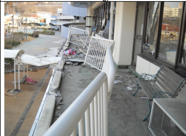
Photo 19: Damage on the second floor deck
