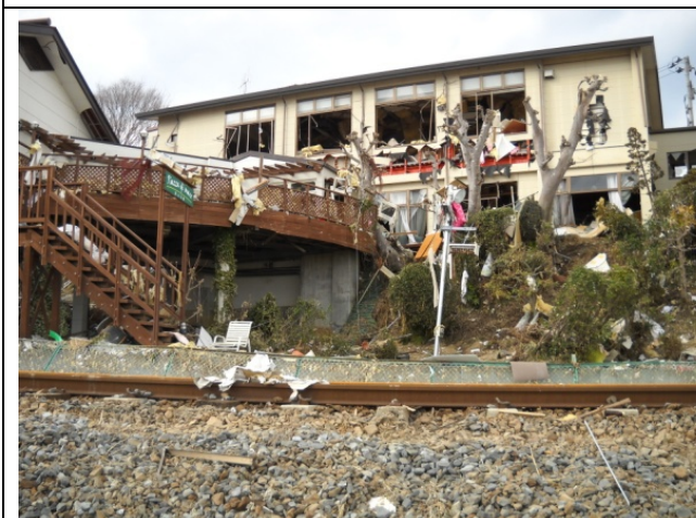
Photo 16: A drive-in building near the shore
