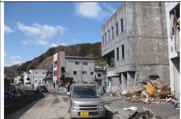
Photo 5: Only timber houses behind an RC building survived from wash away
