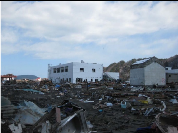
Photo 7: Community Center Building
