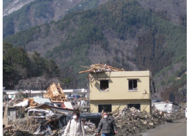
Photo 6: RC or concrete block masonry buildings are left standing
