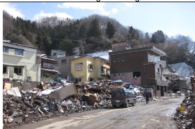
Photo 5: Only timber houses behind an RC building survived from wash away
