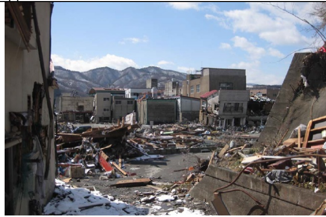
Photo 3: Higashimae-machi, Kamaishi City, approx. 170 from the harbor. Timber houses did not maintain their original configuration.
