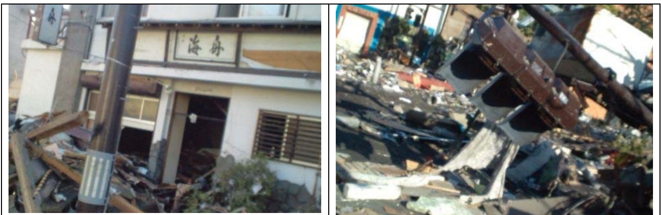
Photo 1: 3-chome (Aoba Street), Kamaishi City, approx. 560 m from Kamaishi Harbor
