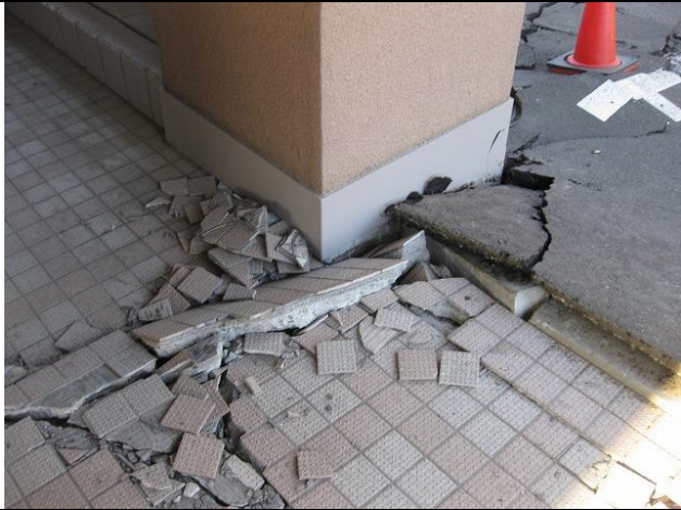
Photo 19: Damage at the base of a first-story column
