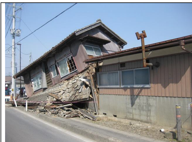
Photo 2: Collapse of a two-story timber house
