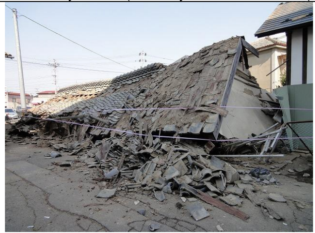
Fig. 7: Collapse of a Godown, adjacent to Ohsaki City Municipal Building
