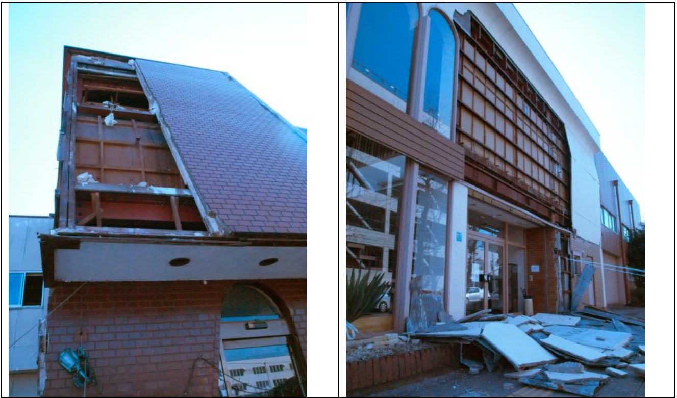
Photo 14: Fall of exterior curtain walls in steel construction
