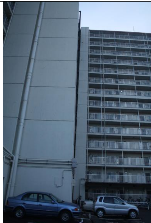
Photo 18: Expansion joint between two buildings (left on March 12, and right on March 16)
