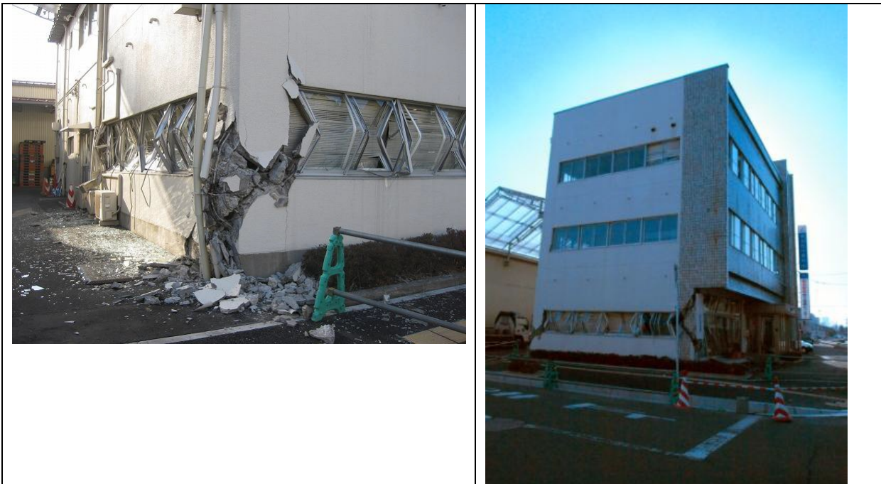
Photo 13: Collapse of a three-story reinforced concrete building in Oroshi-machi 3-chome, Wakabayashi-ku
