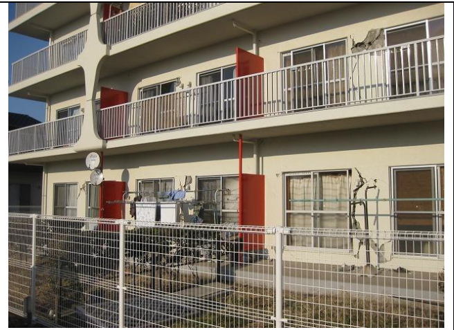
Photo 17: Shear failure of non-structural exterior walls
