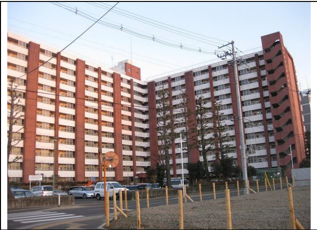
Photo 25: Kohriyama Municipal Apartment Building in Nagamachi, Taihaku-ku
