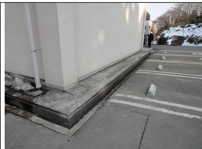
Photo 12: Ground cracking along the periphery of
