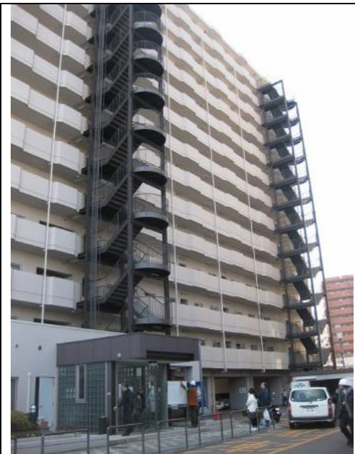
Photo 8 (a) A 14-story reinforced concrete building
