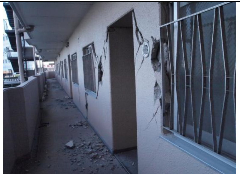
Photo 8 (b): Damage of non-structural walls in the hall way
