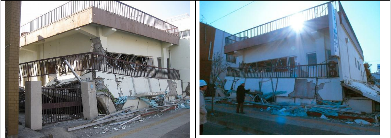
Photo 12: Collapse of a two-story reinforced concrete building in Oroshi-machi 2-chome, Wakabayashi-ku
