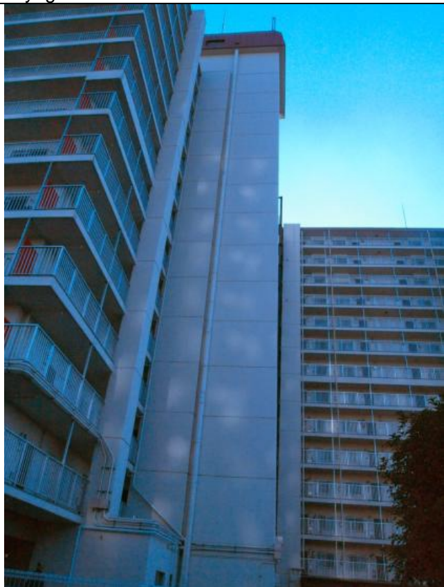
Photo 18: Expansion joint between two buildings (left on March 12, and right on March 16)
