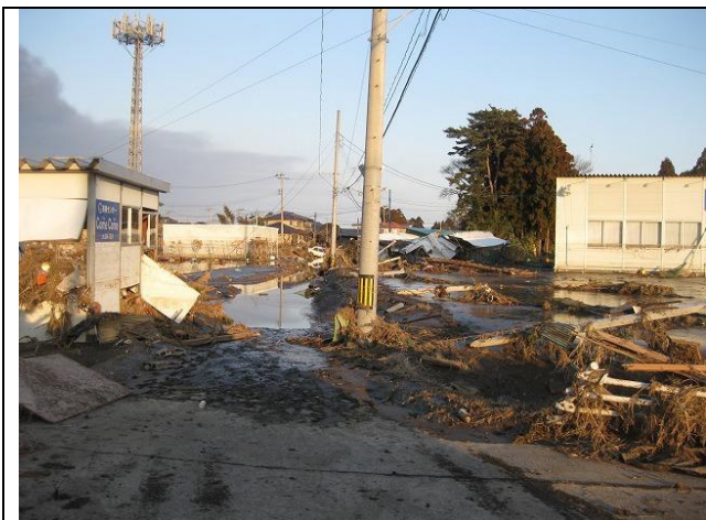
Photo 24: Damage of Gamoh residential area due to tsunamis
