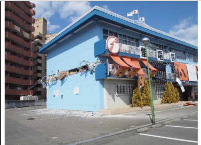
Photo 7: Collapse in the second story
