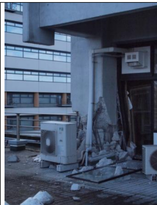
Photo 3: Damage of north-east corner column
