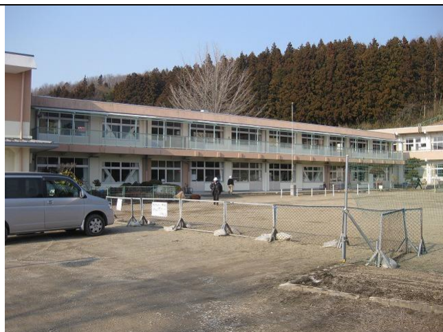
Photo 14: Overview of Uenome Elementary School (No damage)
