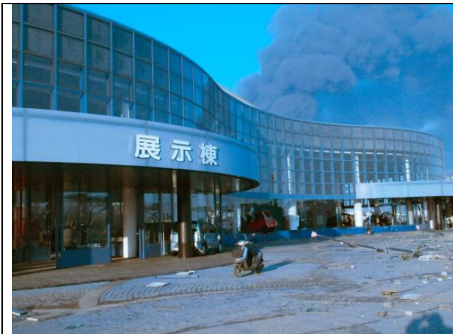
Photo 22: Damage of Miyagi Yume Messe by tsunami
