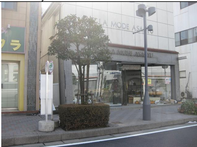
Photo 8: A tilted two-story house for combined use for shop and residence
