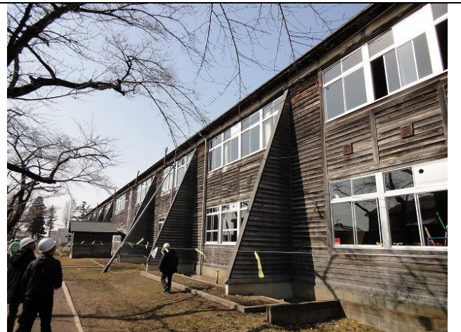
Photo 5: Ohsaki City Municipal Furukawa No.1 Elementary School (two-story timber construction)
