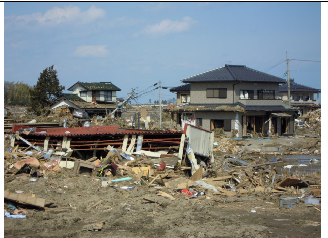
Photo 12: Tsunami water reached the first story roof
