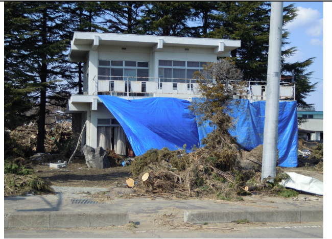
Photo 10: A reinforced concrete house is standing although the first story was attacked by tsunami waves
