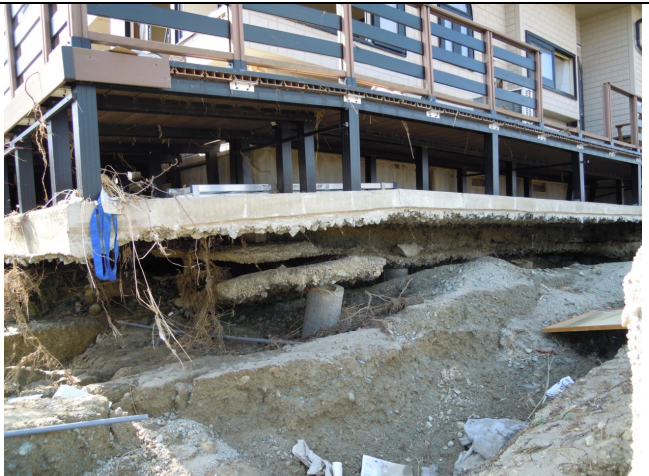
Photo 6: Pile foundation, which implies poor soil conditions in this area
