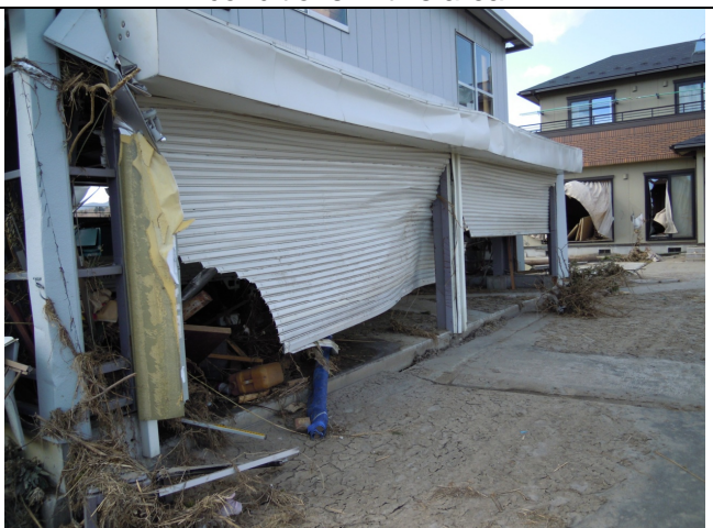
Photo 8: Rolling door shutter was broken, and tsunami water went inside the building
