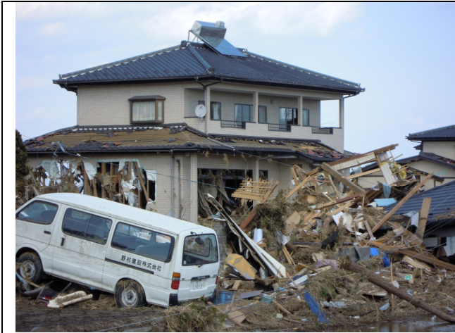
Photo 3: Contents of the first story rooms were washed away and emptied by tsunami waves
