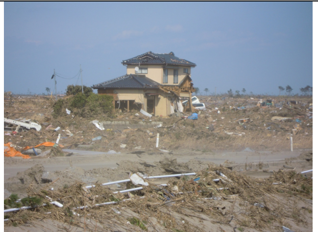
Photo 4: First story is about to collapse during tsunami attacks
