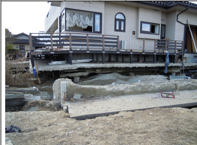
Photo 5: Foundation was exposed by tsunami wave wash
