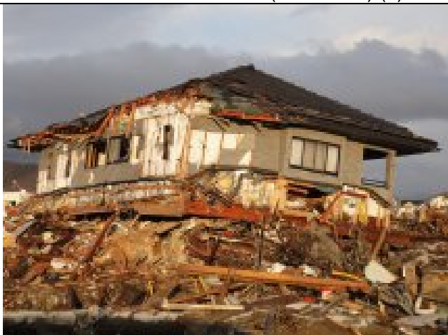
Photo 41: Minami-Hama area; a timber house moved by tsunami waves
