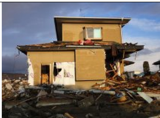
Photo 44: Minami-hama area; a timber house standing (1)
