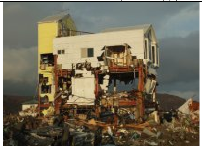
Photo 42: Minami-hama area; a steel construction
