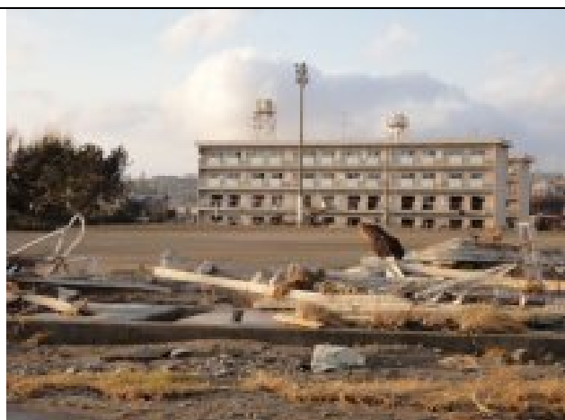
Photo 50: Minami-hama area; Minami-hama apartment building
