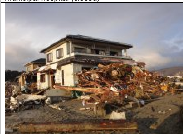
Photo 45: Minami-hama area; a timber house standing (2)
