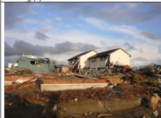
Photo 47: Minami-hama area; steel construction
