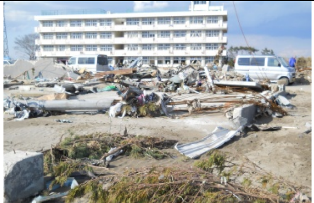
Photo 12: Overall view of the Sendai Municipal Arahama Elementary School; tsunami wave submerged the lower two stories.
