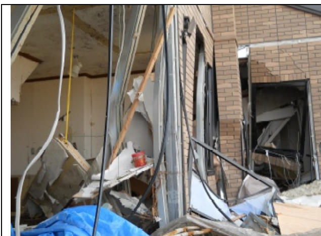
Photo 17: Close up view of the building shown in Photo 14 (3).
