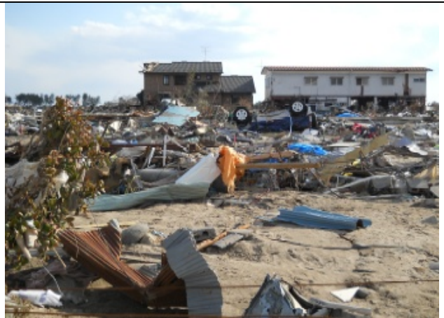
Photo 14: Steel construction remained standing in Arahama District
