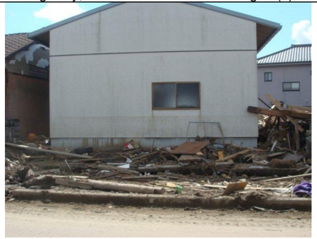
Photo 4: Tsunami wave reached the roof of the building although the building was not damaged.
