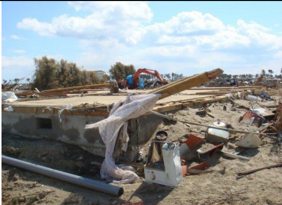
Photo 11: A house was completely washed away except for the foundation (2).
