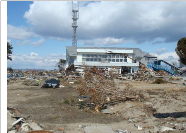
Photo 13: Gymnasium of the Arahama Elementary School; tsunami water flooded inside to yield complete damage to the content.
