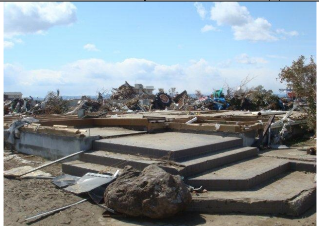
Photo 10: A house was completely washed away except for the foundation (1).
