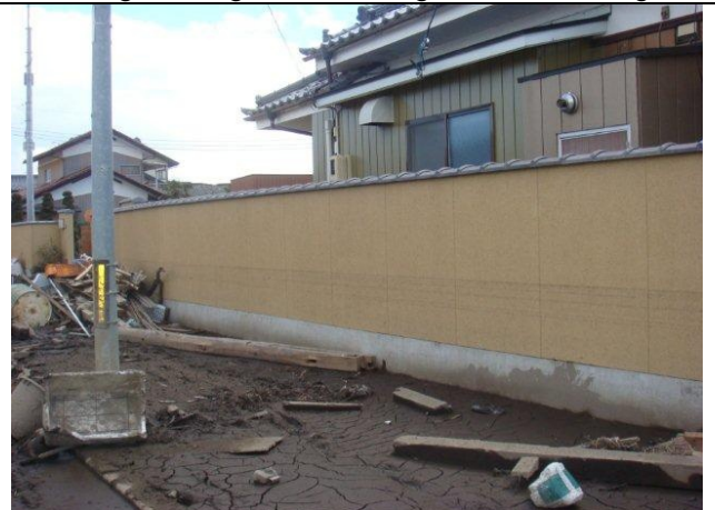
Photo 6: No damage was observed to the concrete block masonry walls
