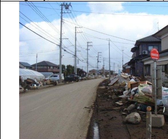
Photo 3: Roads have been cleared
