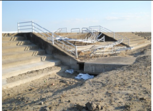
Photo 20: Damage of rails on the embankment (1).
