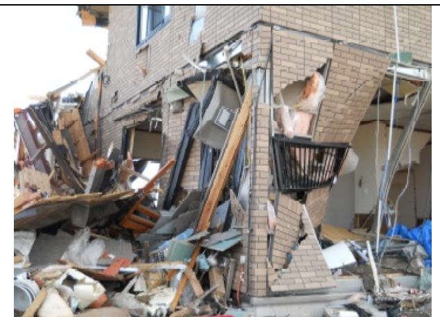
Photo 16: Close up view of the building shown in Photo 14 (2).
