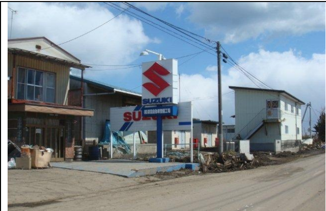
Photo 1: Outflow items beyond the Sendai Tobu Highway; but houses were not damaged (1)
