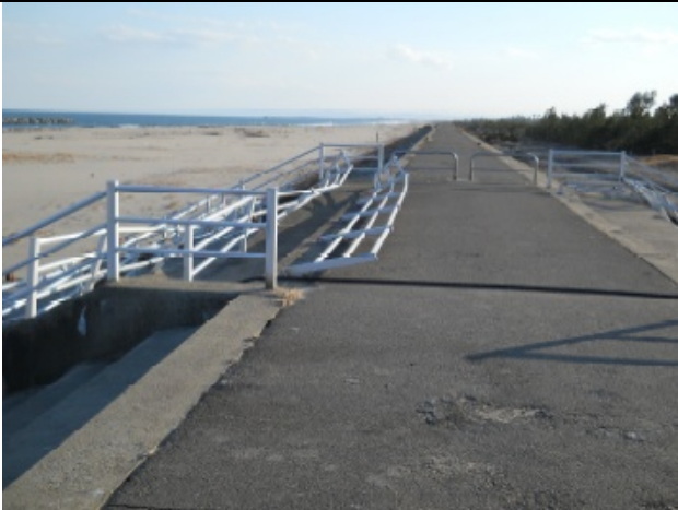
Photo 21: Damage of rails on the embankment (2).
