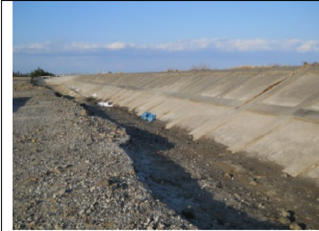
Photo 19: Undamaged Breakwater embankment
