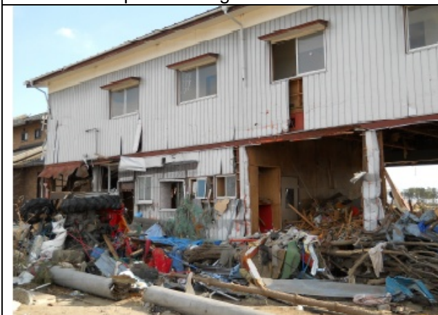
Photo 15: Close up view of the building shown in Photo 14 (1).
