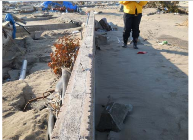
Photo 6: All anchor bolts on the surface of foundation were bent in the direction normal to the coast line.
