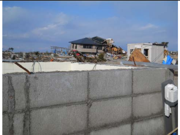
Photo 8: The bent direction of anchor bolts and face direction on outflow materials coincided.
