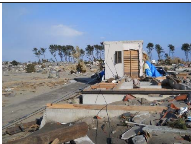
Photo 13: West side of Building A, approximately 900 m from the coast.
