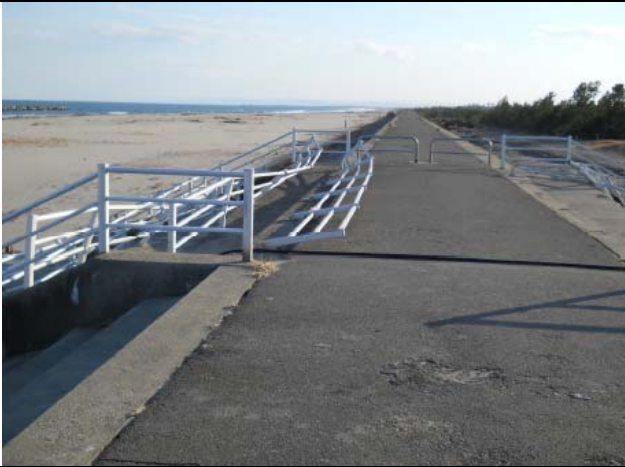
Photo 1: Hand rails on the embankment suffered no damage in the direction parallel to the tsunami wave and heavy damage normal to the wave.
