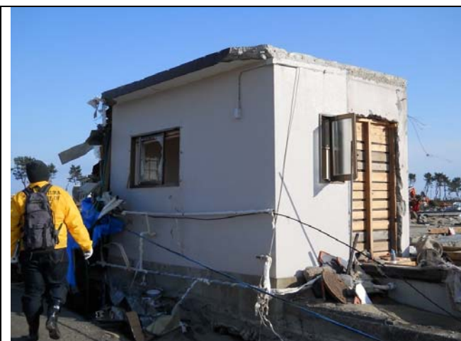
Photo 12: North side of Building A
