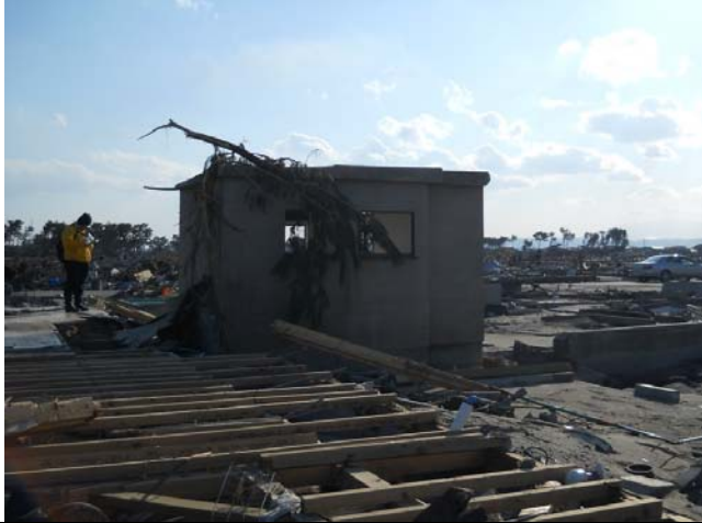
Photo 14: North side of Building B; approximately 900 m from the coast
