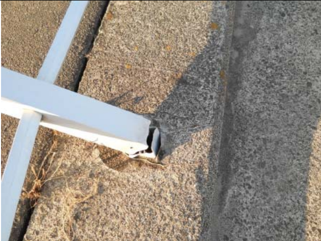
Photo 3: The fracture at the base of a hand rail.
