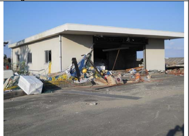
Photo 17: South side of Building C, approximately 400 m from the coast.
