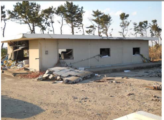
Photo 16: East side of Building C, facing to the tsunami flow.
