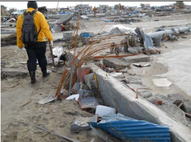
Photo 5: All electric poles fell in the same direction, normal to the coast line.
