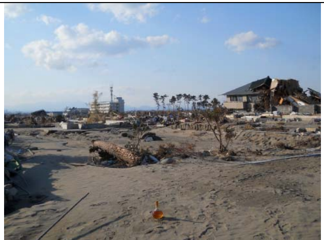
Photo 10: Tsunami wave reached the second floor of a steel skeleton house.
