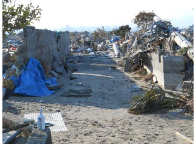
Photo 4: All electric poles fell in the same direction, normal to the coast line. Concrete block masonry wall normal to the tsunami flow did not fail.
