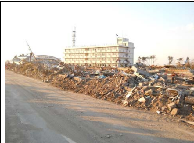
Photo 9: Tsunami wave height was estimated to be 4 m at Arahama Elementary School.
