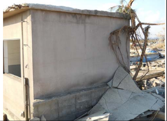
Photo 15: East side of Building B, no opening facing the tsunami flow.
