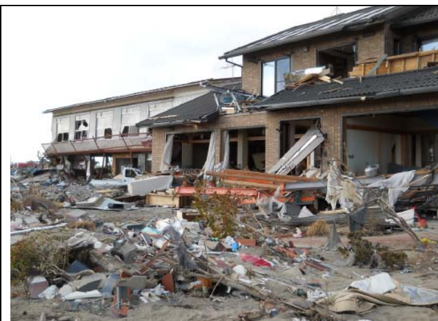
Photo 11: Tsunami wave reached the second floor of a steel skeleton house.
