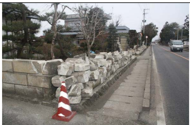
Photo 5: Fall of masonry walls
