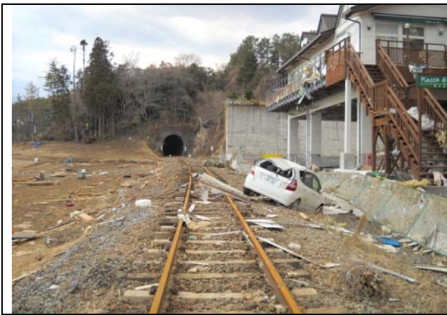
Photo 14: A view toward a tunnel.
