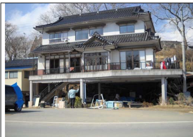
Photo 22: A timber house on one-story reinforced concrete foundation
