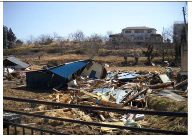
Photo 7: Broken houses in the low land and an untouched house on the hill.
