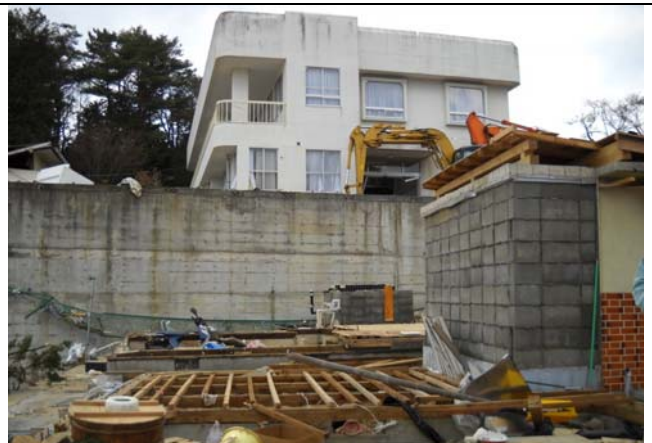
Photo 19: A timber house was washed away leaving the foundation, next to the warehouse.
