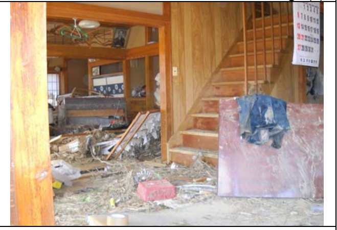
Photo 4: Inside of a house inundated by water.
