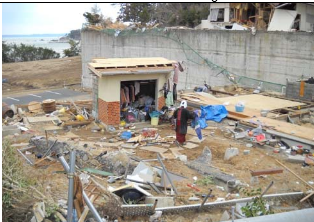
Photo 18: A concrete block warehouse below the hotel building
