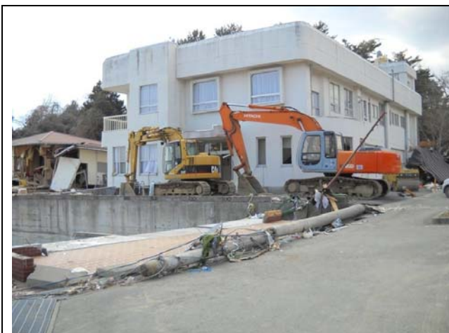
Photo 20: A two-story reinforced concrete old-age home
