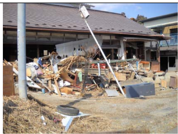
Photo 23: Damaged adjacent timber house
