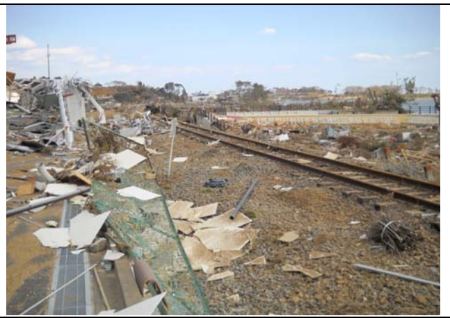
Photo 15: A view from the tunnel side.
