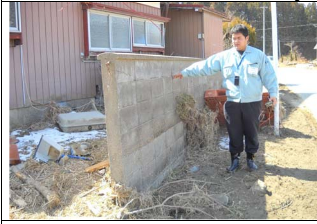
Photo 3: The level of tsunami wave above the floor.
