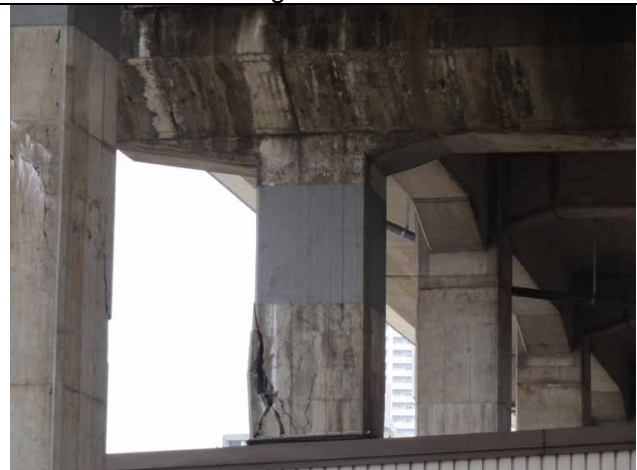
Photo 8: Shear failure of a pier below the fiber reinforcement retrofit of the Shinkansen Viaduct
