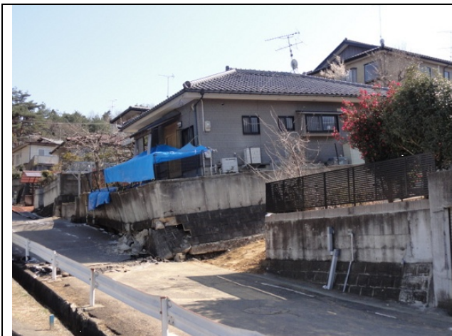
Photo 1: Failure of retaining walls. Oritate 5-chome, Aoba-ku
