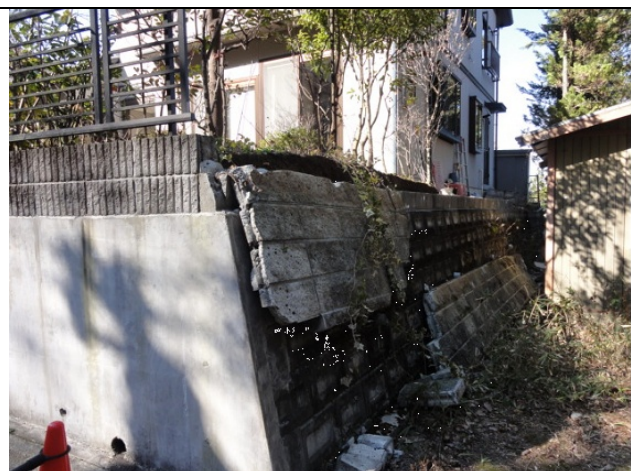
Photo 6: Fall of concrete block walls. Oritate 5-chome, Aoba-ku
