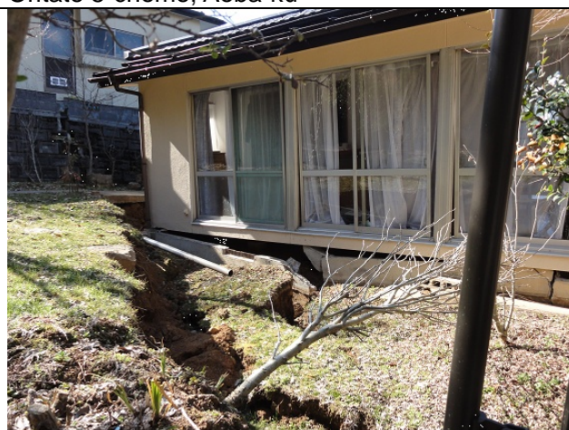
Photo 8: Ground settlement (80 cm).
