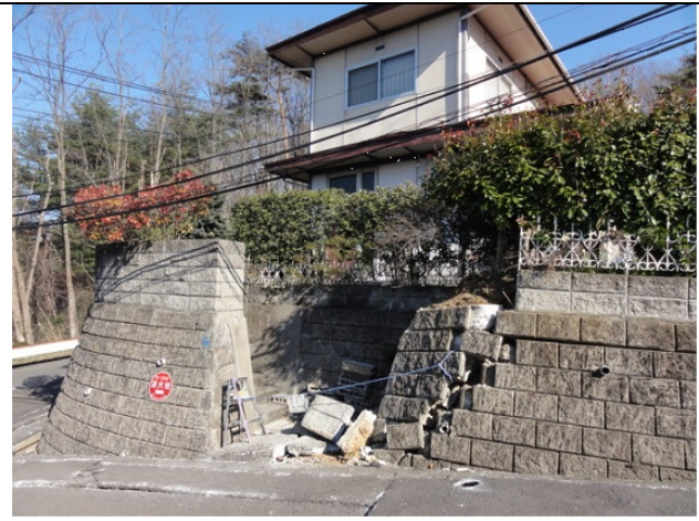
Photo 14: A house of relatively light damage in this area
