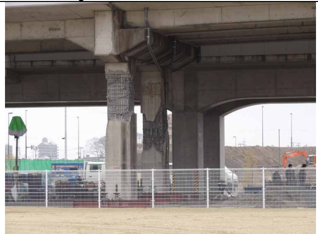
Photo 6: Piers of viaducts for the Shinkansen (built in 1982) and the Tohoku Line (built in 2006)
