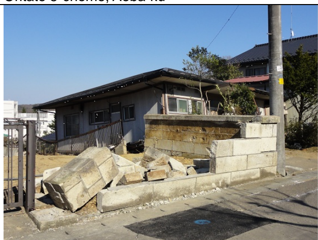
Photo 7: Fall of masonry walls and damage of a house due to land slide Oritate 5-chome, Aoba-ku
