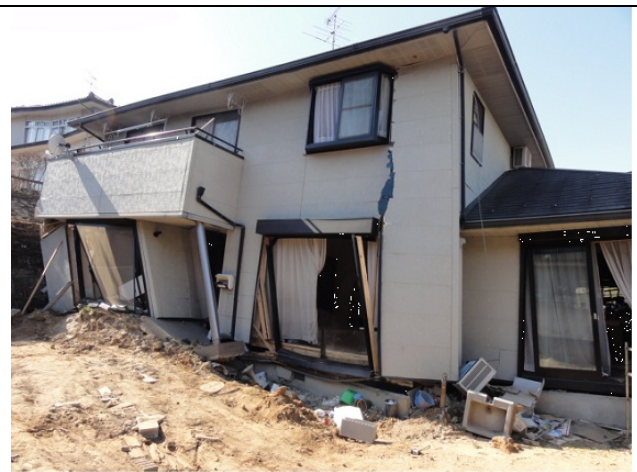
Photo 2: Damage of a house caused by land slide. Oritate 5-chome, Aoba-ku
