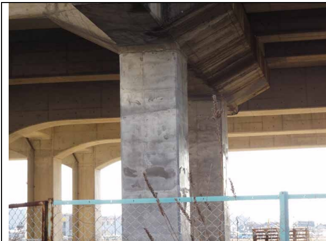
Photo 9: Shinkansen Viaduct, repair work of a pier after the shear failure to the core concrete.
