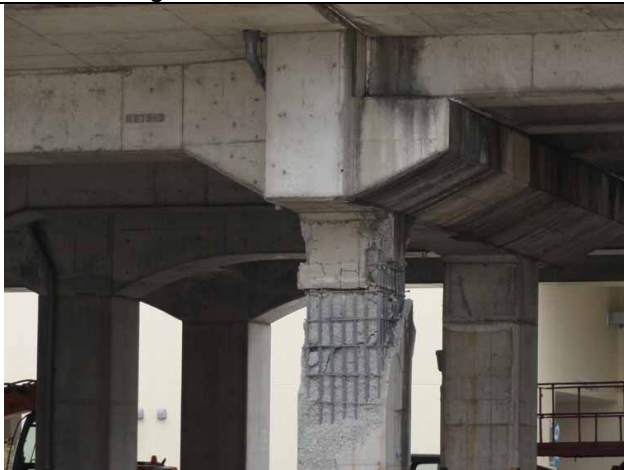
Photo 5: Viaduct of the Shinkansen Line, shear failure penetrated to the concrete core of the pier.
