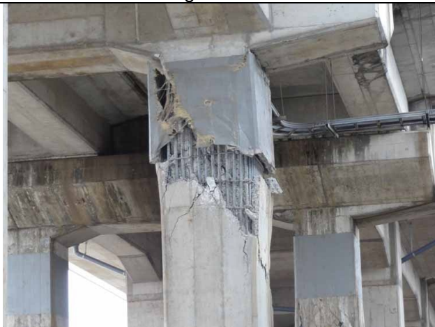
Photo 7: Fracture of retrofit fiber reinforcement sheet of a pier of the Shinkansen Viaduct
