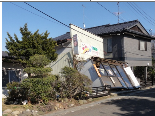
Photo 9: Damage of a house due to land slide. Oritate 5-chome, Aoba-ku
