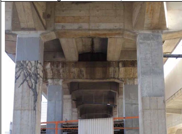
Photo 11: Shinkansen Viaduct, right pier after the fracture of fiber reinforcement sheet (see Photo 9), and left pier after shear cracking (see Photo 10).
