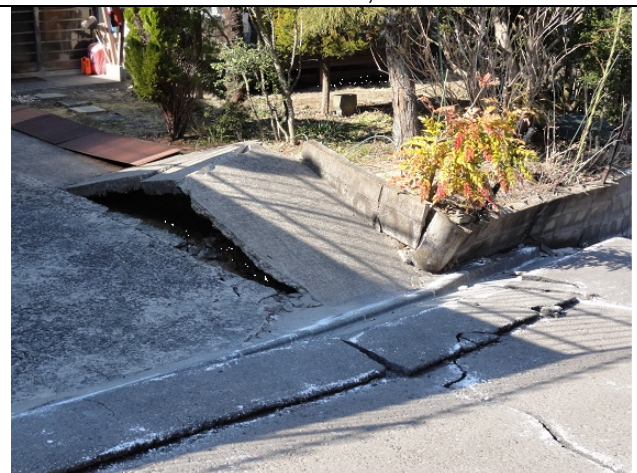
Photo 4: Damage of road surface. Oritate 5-chome, Aoba-ku
