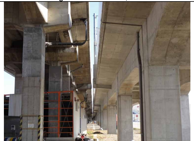
Photo 12: Left is the Shinaknsen (1982) viaducts and right is the Tohoku Line (2006) viaducts
