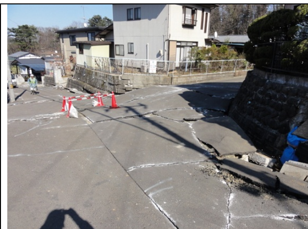
Photo 5: Failure of road surface. Oritate 5-chome, Aoba-ku
