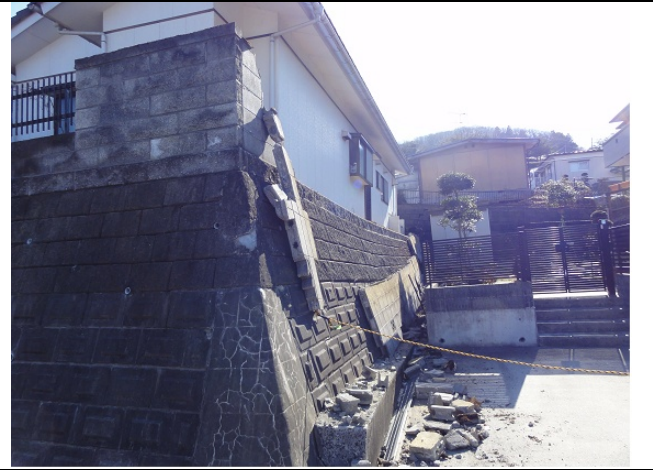
Photo 12: Fall of concrete block walls. Oritate 5-chome, Aoba-ku
