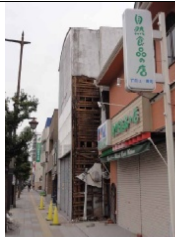
Photo 4: Fall of mortar finishing from a timber house
