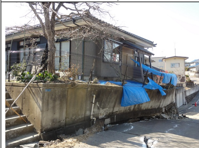
Photo 3: Failure of retaining walls. Oritate 5-chome, Aoba-ku
