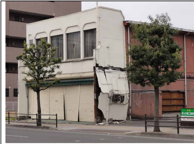
Photo 3: Fall of exterior finishing from a timber house
