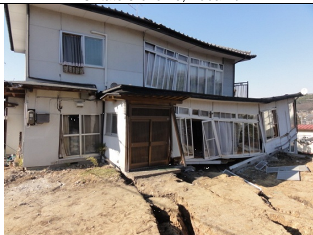
Photo 10: Damage of a house due to land slide Oritate 5-chome, Aoba-ku
