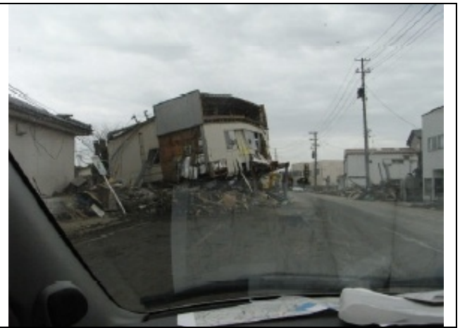
Photo 2: First story was broken.
