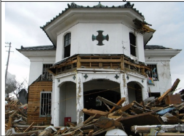
Photo 3: Front view facing the sea.
