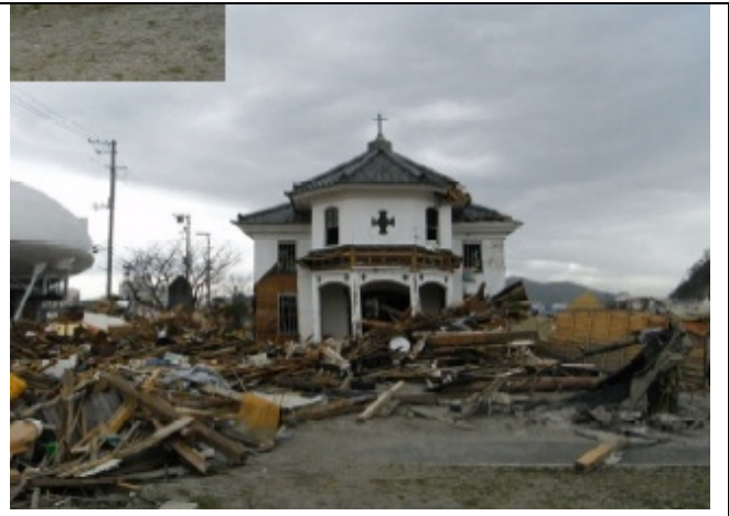
Photo 2: Front view facing the sea.
