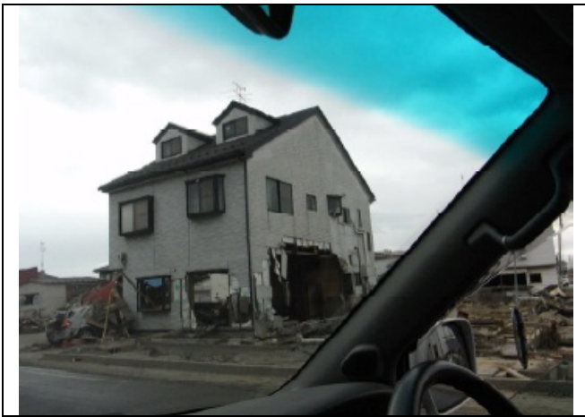
Photo 1: Damage by tsunami.
