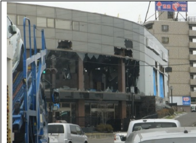
Photo 1: Exterior finishing was damaged by the April 6 aftershock in Sendai City.
