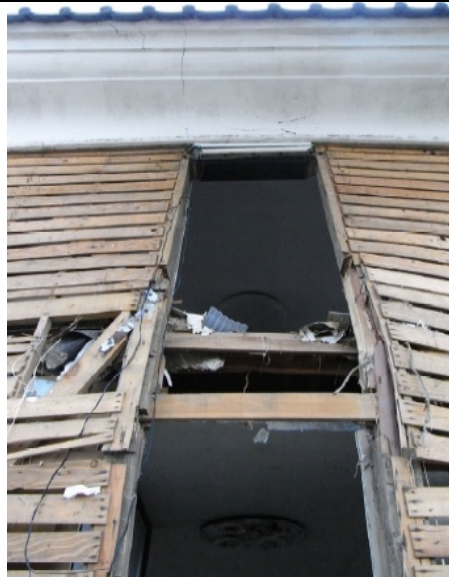
Photo 6: Damage in the back.
