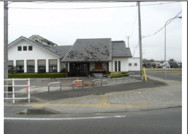
Photo 2: Fall of roof tiles and breakage of window glasses, probably due to the April 7 aftershock.
