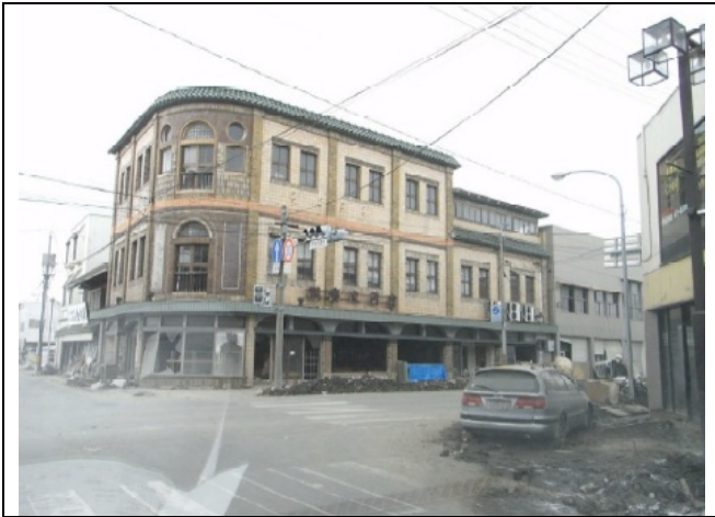
Photo 1: China-ware Kankei-maru, the damage in the first story due to inundation (N o. 4 in route map)
