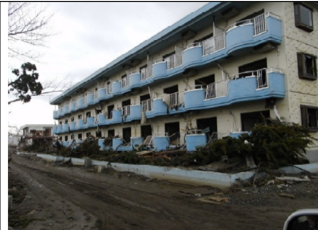
Photo 9: Damage was observed up to the second story (No.1 in route map).
