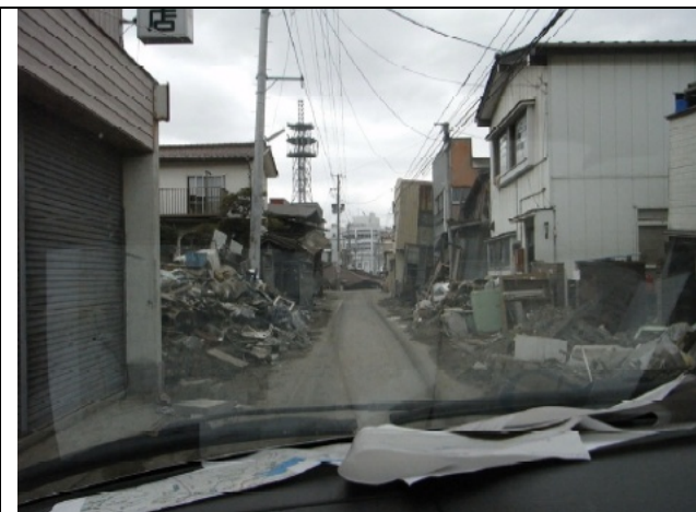
Photo 13: Damage in densely built up area. Roads were not passable (No. 2 in Route Map).
