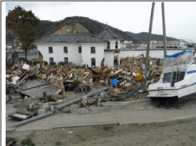
Photo 1: Front view facing the sea.
