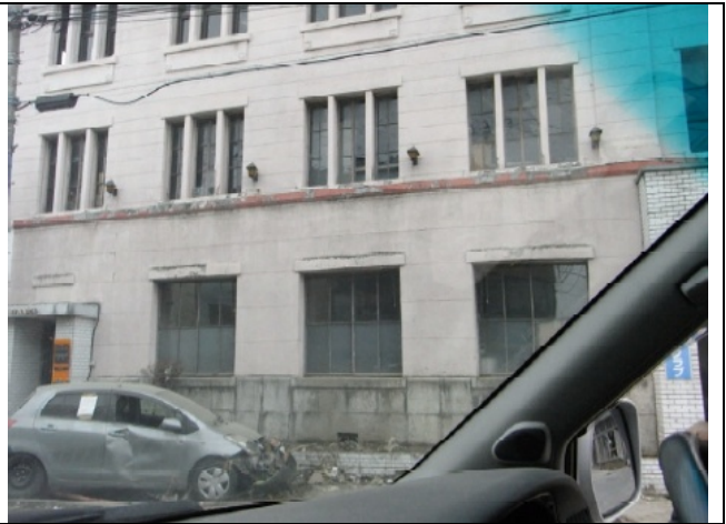
Photo 2: Daini SS building, many buildings suffered damage in the first story due to tsunami.
