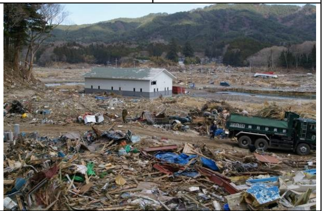
Photo 4: Only remaining building in the neighborhood of the collapsed breakwater.
