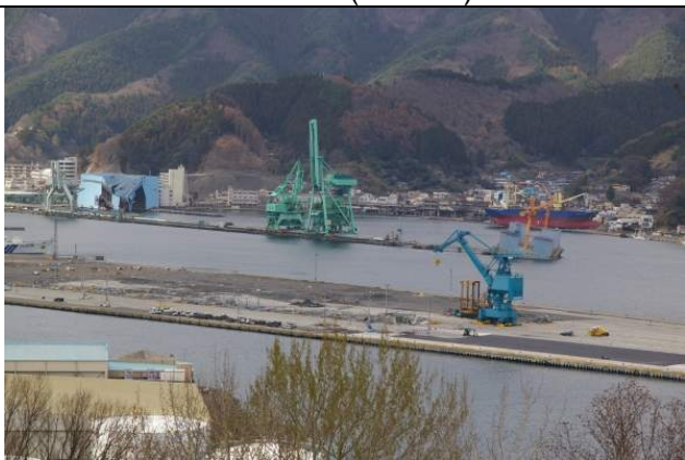
Photo 3: Kamaishi Port. Grounding of a large scale ship.
