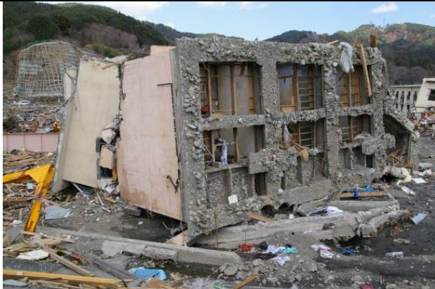
Photo 3: The foundation of the apartment building shown in Photo 2.
