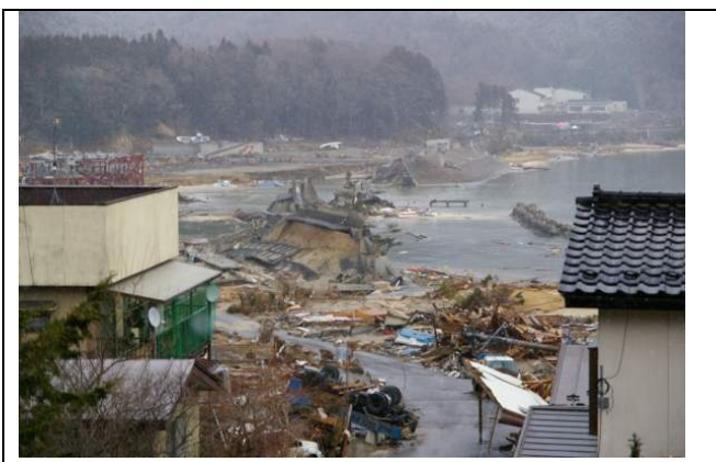
Photo 1: Collapsed breakwater (On March 23).
