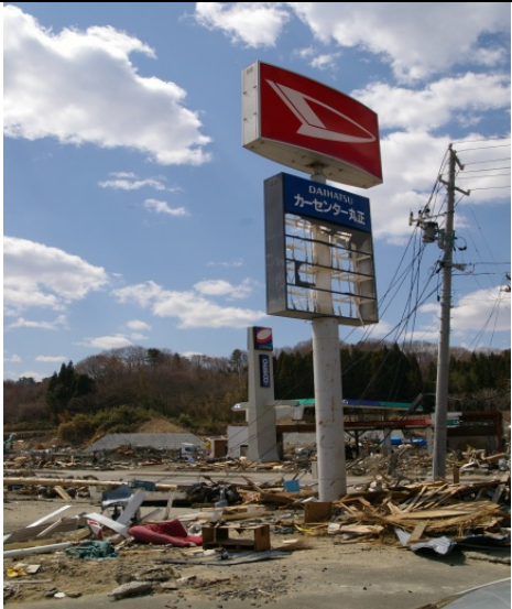
Photo 3: Damage of signboard. Some indication of tsunami height.
