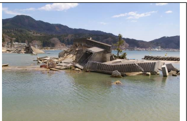
Photo 2: Collapsed breakwater
