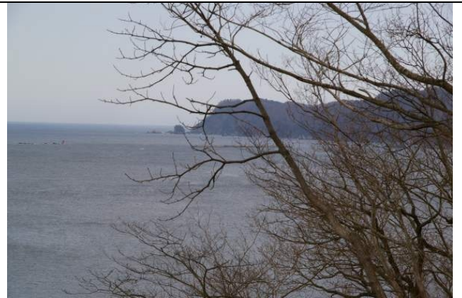
Photo 2: View of collapsed Kamaishi Port Mouth Sea Wall (right side).
