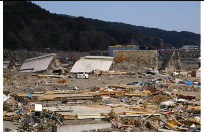
Photo 4: Overturned and dislocated breakwater by tsunami.
