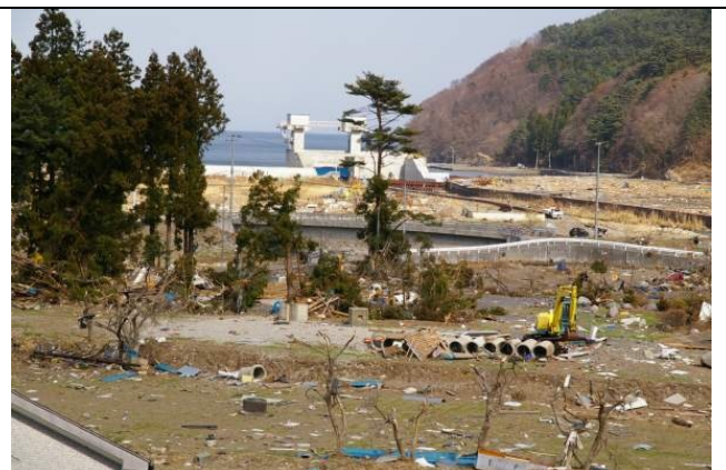
Photo 2: A brand new water gate. Houses were all washed away.
