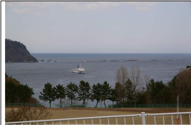
Photo 1: View of collapsed Kamaishi Port Mouth Sea Wall (left side)
