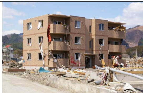
Photo 6: A reinforced concrete building standing, completely submerged under water.
