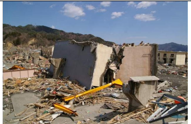
Photo 2: An overturned two-story reinforced concrete apartment building.
