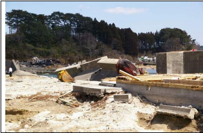
Photo 3: Collapsed breakwater.
