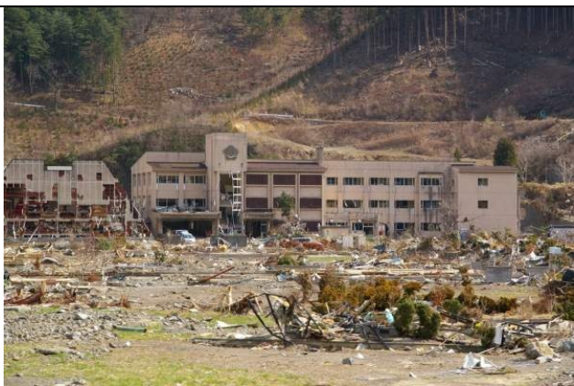
Photo 1: Toni Elementary School. Tsunami reached the third floor of the building.
