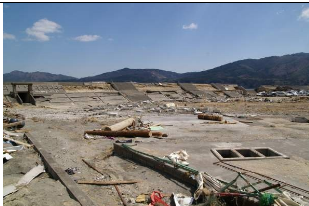
Photo 1: View of breakwater. The tsunami wave flowed over the breakwater.
