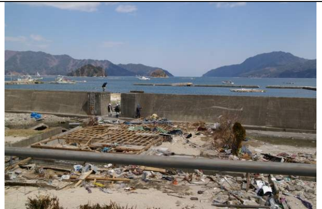
Photo 2: Remaining parts of breakwater.
