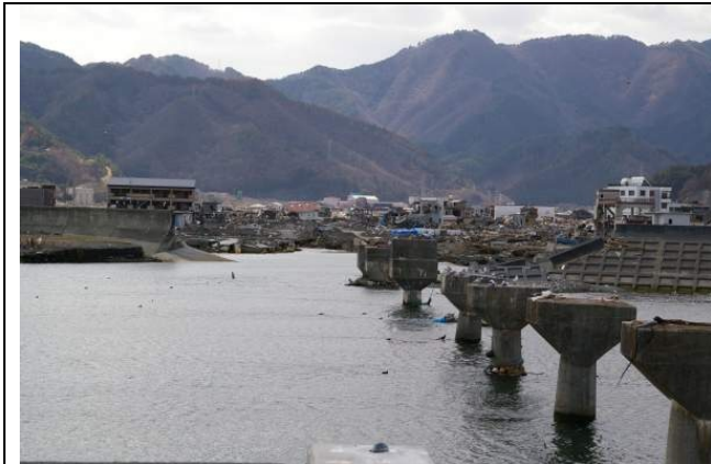
Photo 1: Breakage of embankment, view toward Ohtsuchi station. Front structure is washed away piers of railway bridge of the Yamada Railway Line.
