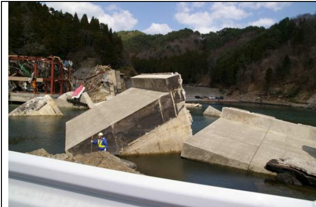
Photo 1: Failure of breakwater.
