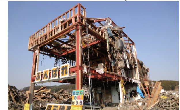
Photo 10: The steel skeleton of a commercial building remained; exterior walls and roofs were washed away.
