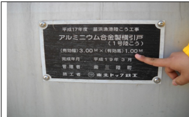
Photo 1: 1-m high tidal embankment with sliding door was constructed, but of no use.
