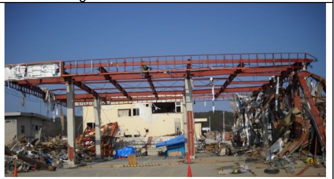
Photo 9: The steel skeleton of a gas station building remained; washed away rubbish stayed on the beams and columns on the right.
