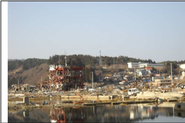
Photo 24: Sea water could not be drained due to ground settlement. High tide repeatedly flood the area. The school on the hill did not suffer damage.
