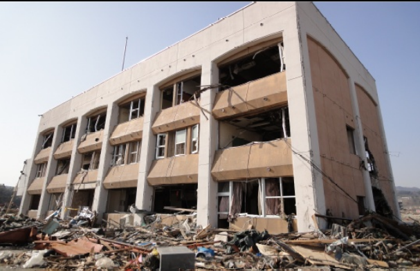
Photo 16: Minami-Sanriku Police Station building (reinforced concrete). The inside is filled with rubbish, and a hole was made in the right side wall by colliding objects.
