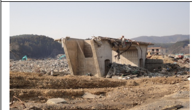
Photo 8: The JR Kesen-numa line. Piers were standing but the railway was washed away and the Shidukawa station was destroyed.
