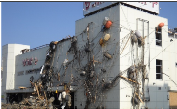
Photo 3: Tsunami wave reached the fourth floor of a reinforced concrete super-market building; washed way fishery nets hang on the building; according to the area residents, many people were saved on the roof.
