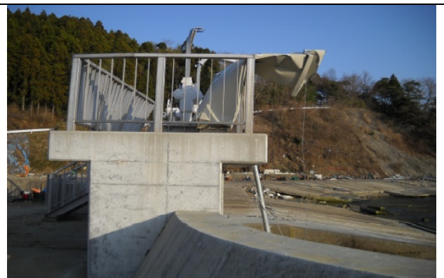
Photo 2: Tsunami wave passed over the tidal embankment and caused the damage.
