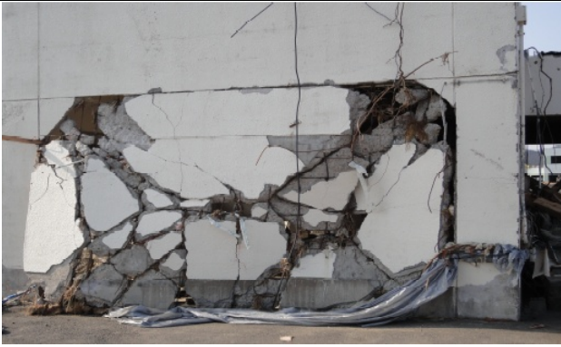
Photo 20: The exterior wall shown in Photo 19.
