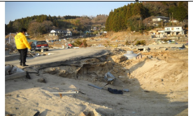
Photo 4: Road side was washed and dangerous for use.
