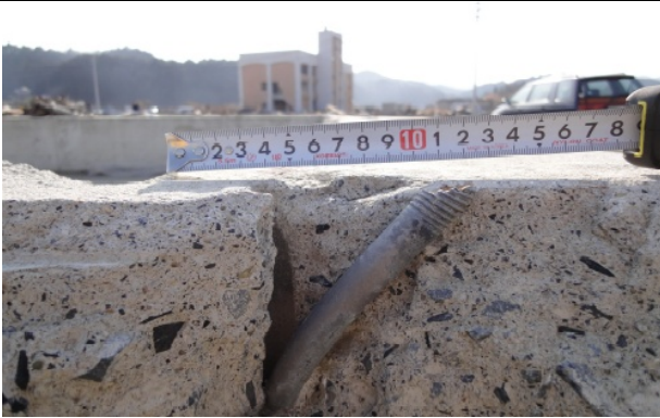
Photo 14: Anchor bolts in the foundation was bent in the direction of tsunami flow.
