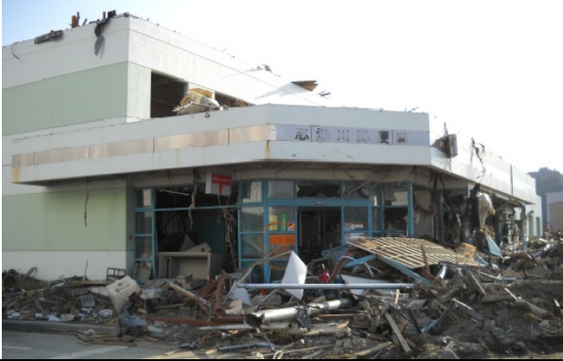
Photo 18: The inside of Shidukawa Post office building (reinforced concrete) was filled with wash away rubbish.
