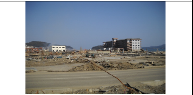
Photo 7: Reinforced concrete condominium and two-story buildings remained standing; skeletons of steel buildings on the left.
