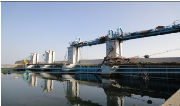
Photo 1: Flood gates were closed at the time of tsunami, tsunami wave passed over the girder for winding gates (blue color).
