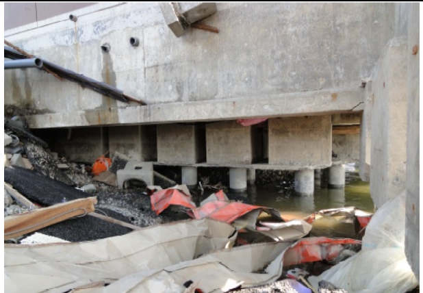
Photo 22: The foundation of a four-story reinforced concrete condominium building near the sea shore; the foundation is exposed.
