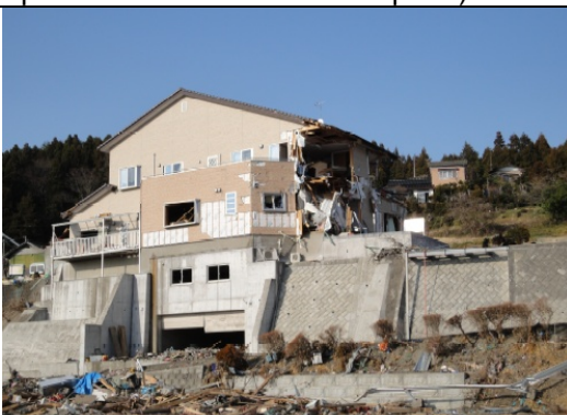
Photo 4: Tsunami passed over 6-m high retaining walls and damaged the houses on the higher level.
