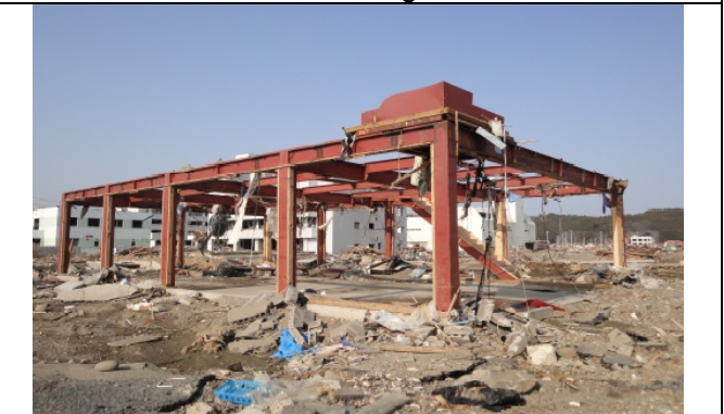
Photo 11: Steel skeleton of a steel building remained.
