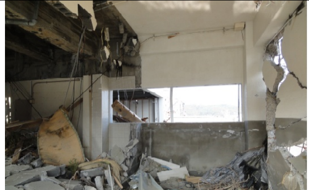
Photo 21: The condition and damage of an interior wall of the building shown in Photo 19.
