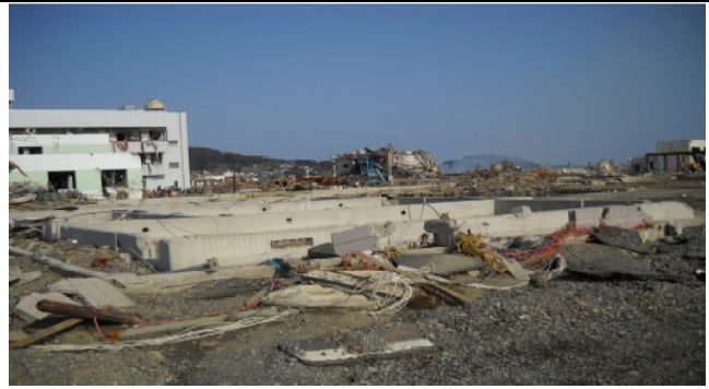
Photo 13: The foundation of a timber house remained at the site. Most houses in Shiomi-cho district showed similar conditions.
