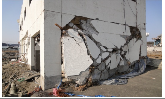
Photo 19: Damage of an exterior wall of a two-story reinforced concrete building; washed away objects must have hit the wall.
