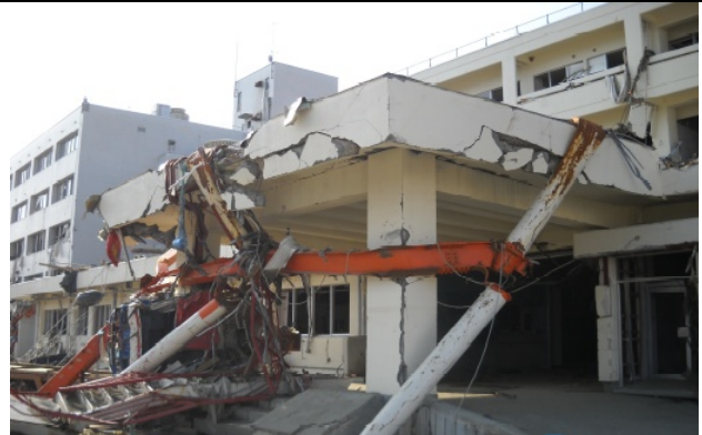
Photo 17: The damage appeared small from the external observation of Shidukawa Hospital (reinforced concrete), but the entrance porch was struck with diameter 300 mm steel columns and H-300x500 section.
