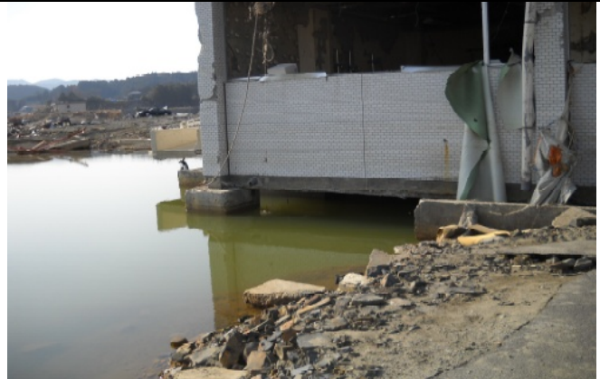
Photo 23: The ground settlement developed muddy puddle.
