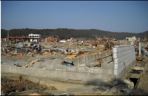
Photo 12: Concrete block walls fell in the direction of tsunami wave flow.
