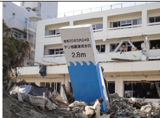
Photo 2: Tsunami wave reached the third floor of the reinforced concrete Shidukawa Hospital building (front panel says the tsunami of the 1960 Chilean Earthquake reached 2.8 m at the point).
