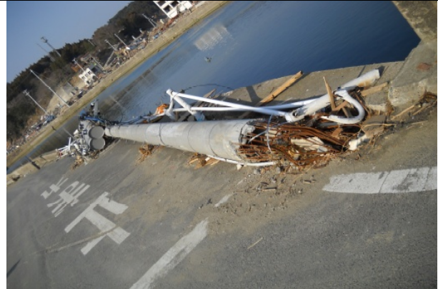
Photo 15: Utility poles fell down in the direction of tsunami flow.
