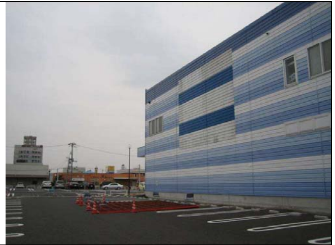
Photo 12: Fall of exterior panel to parking lot
