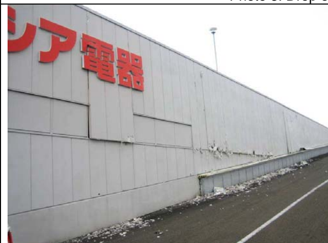
Photo 4: Breakage of ALC (autoclaved light-weight concrete) panel (Building 2)
