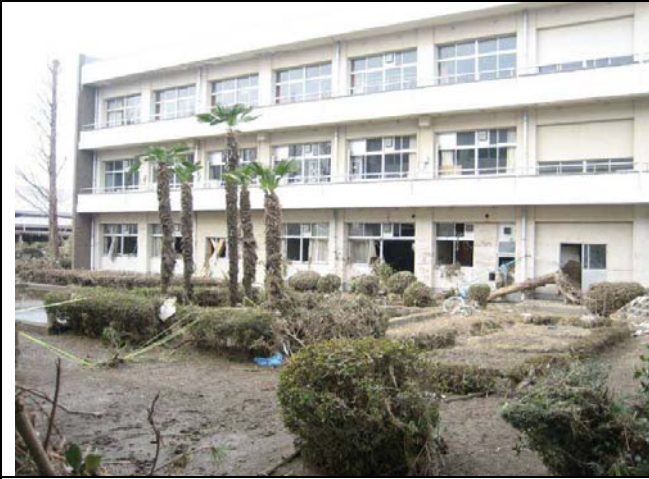
Photo 5: South face of the North Building
