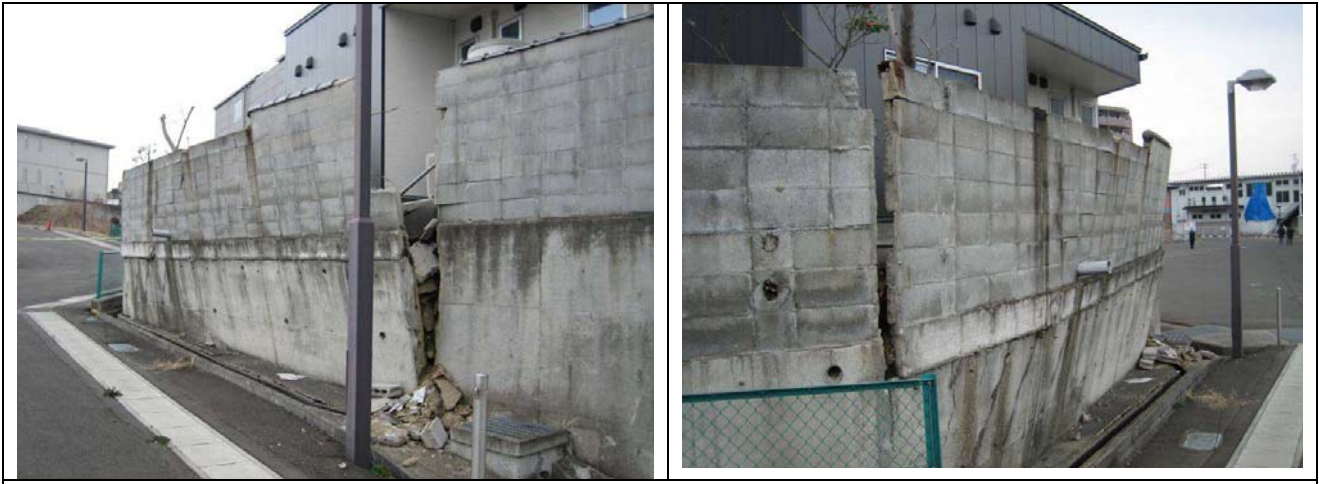
Photo 5: Fall of concrete block walls in the neighborhood
