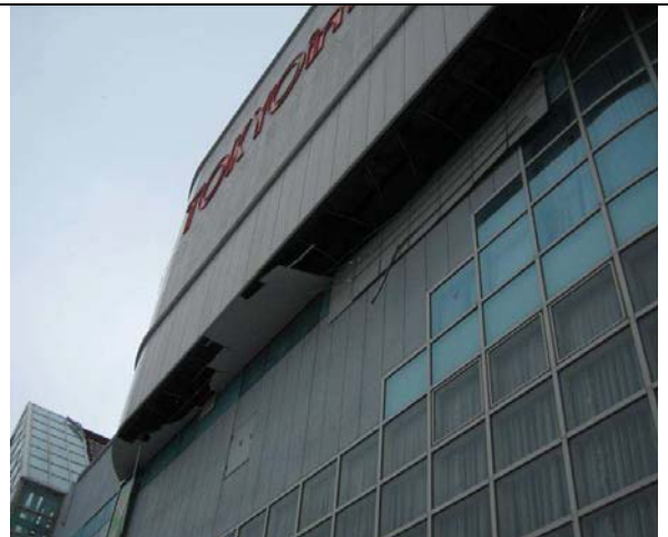
Photo 2: Fall of ceiling (Building 1)
