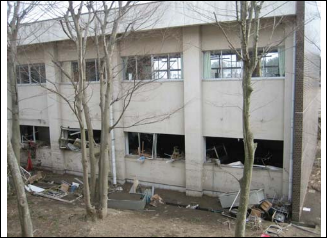
Photo 6: North face of the North Building
