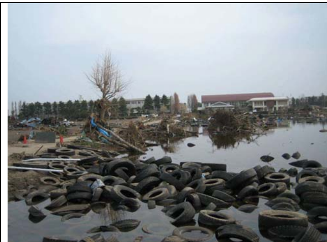
Photo 1: Campus after the tsunami attack
