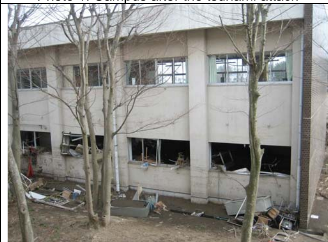
Photo 3: Broken windows in the 1-st story (north face of the South Building)
