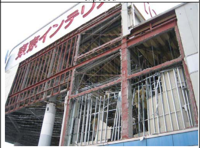
Photo 4: Fall of exterior curtain walls
