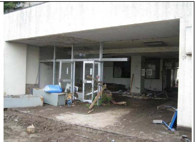
Photo 2: Entrance damaged by the tsunami
