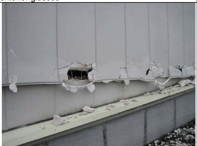
Photo 4: Breakage of ALC (autoclaved light-weight concrete) panel (Building 2)
