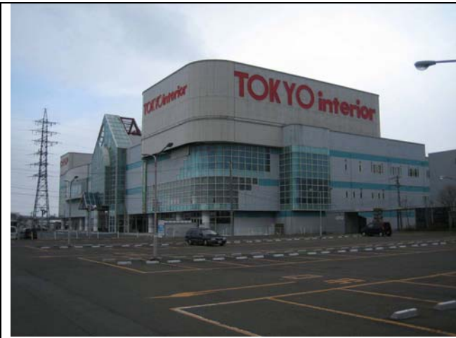
Photo 1: Exterior overall view of Building 1
