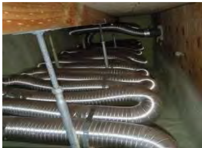
Fig 28: Fresh air in duct will be heat changed by the exhaust air
