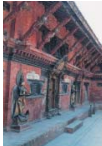
❖ Embellished struts supporting the eaves, southern side of the of quadrangle, the Mul Chok
